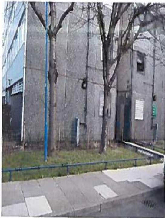
View 3: Subject site Side and Front Elevations
