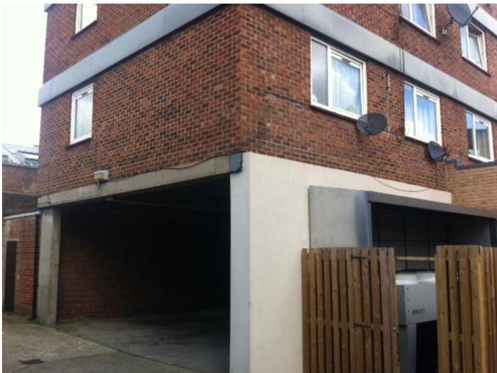
Image 3: Nearest residential positioned at first floor level above acoustic canopy
