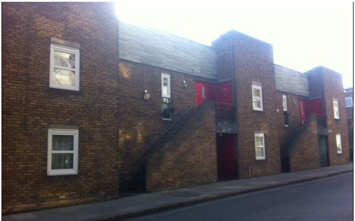
Image 4: Nos. 150-158 Offord Road adjacent site with existing UPVC windows (also Barnsbury Conservation Area)
