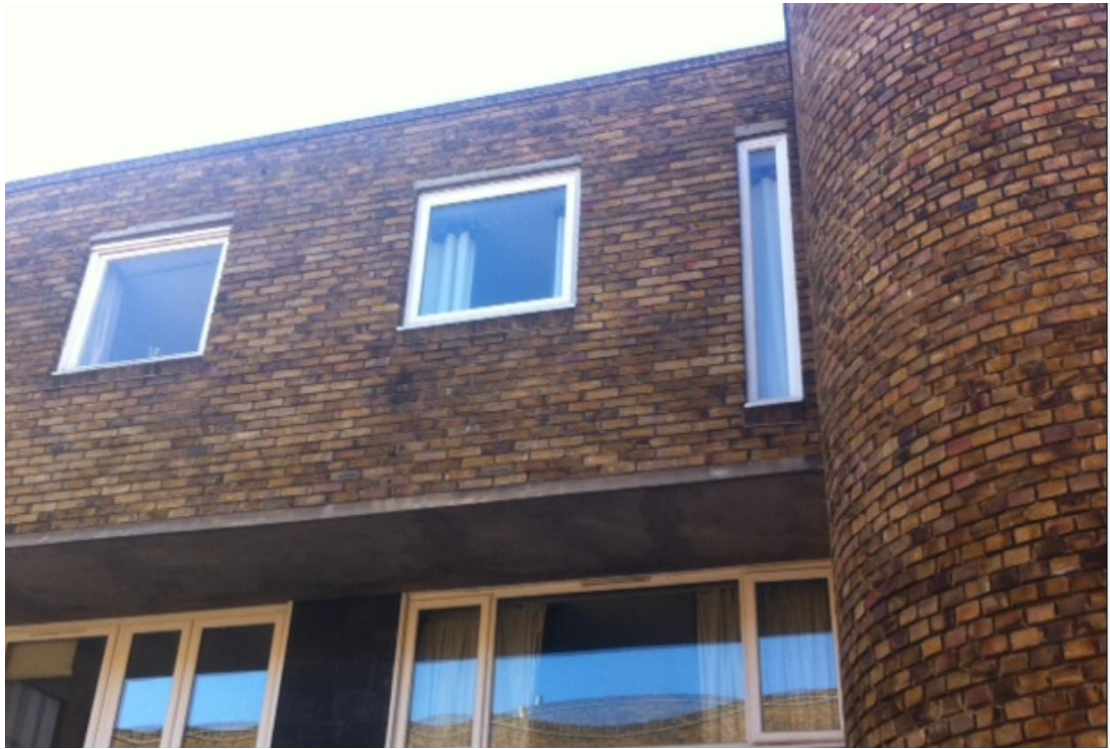
Image 7: Existing variation to window frames in Legion Close with Aluminium, Timber and UPVC
