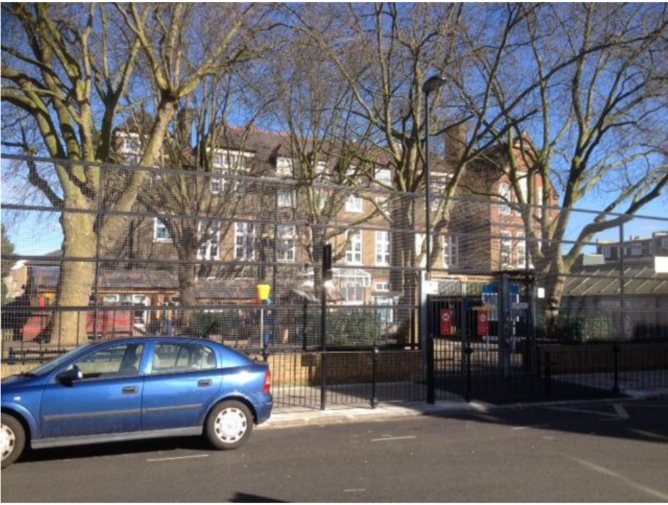
Photo 1 The site looking south east across Sussex Way
